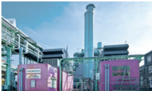
01 | Gas turbine plant, Infracore Höchst.
